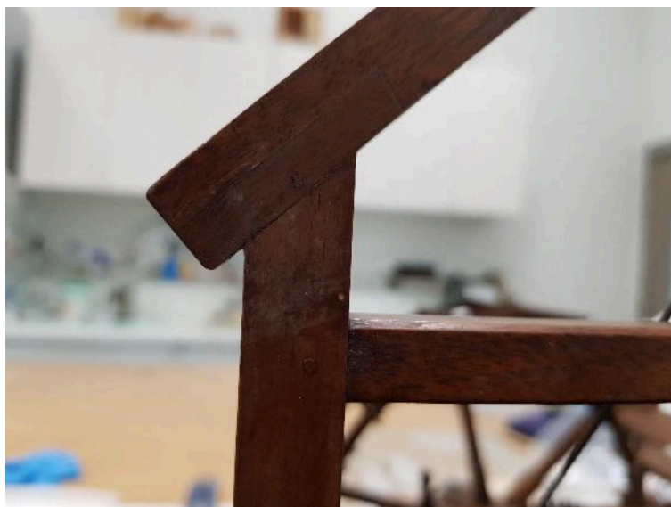
Figure 11 Assemblages tenon-mortaise chevillés
